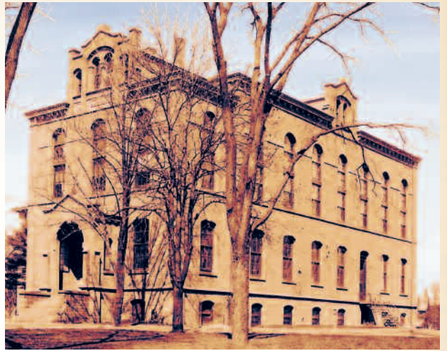
Geological Hall (1872) , Hardenbergh's first complete commission, was built of stone rather than the expensive brick Hardenbergh had specified.
